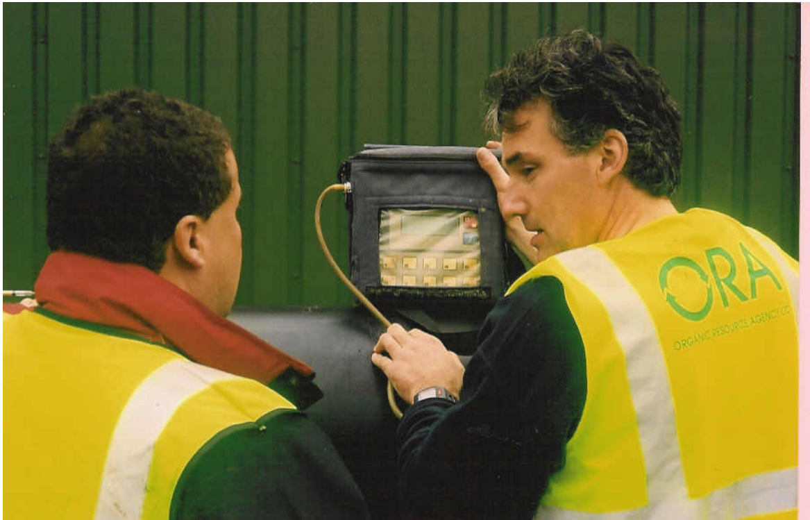
Plate 3. Assessment of exhaust air going to the scrubber and biofilter
